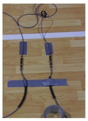
**Step 5:** At the center of the strip, tape down the cables as shown. Each cable is taped down over the rubber-reinforced section of the cable. This is the section of cable that will flex and the rubber hose provides additional strain relief.
